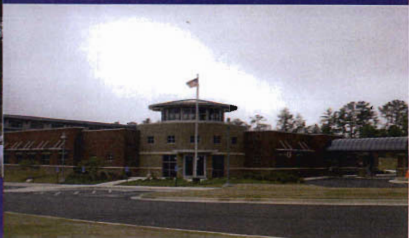
Below: The Bailey-Alexander Water and Sewer complex houses field operations, administration and billing services.
